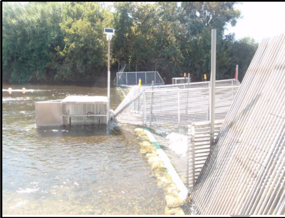
Figure 9. Modifications to the 2010 Tuolumne River weir included the removal of approximately a nine foot section of the substrate rail and weir panels at the location of the passing chute, removal of the live box, and creation of a small funnel to direct fish into the passing chute.
