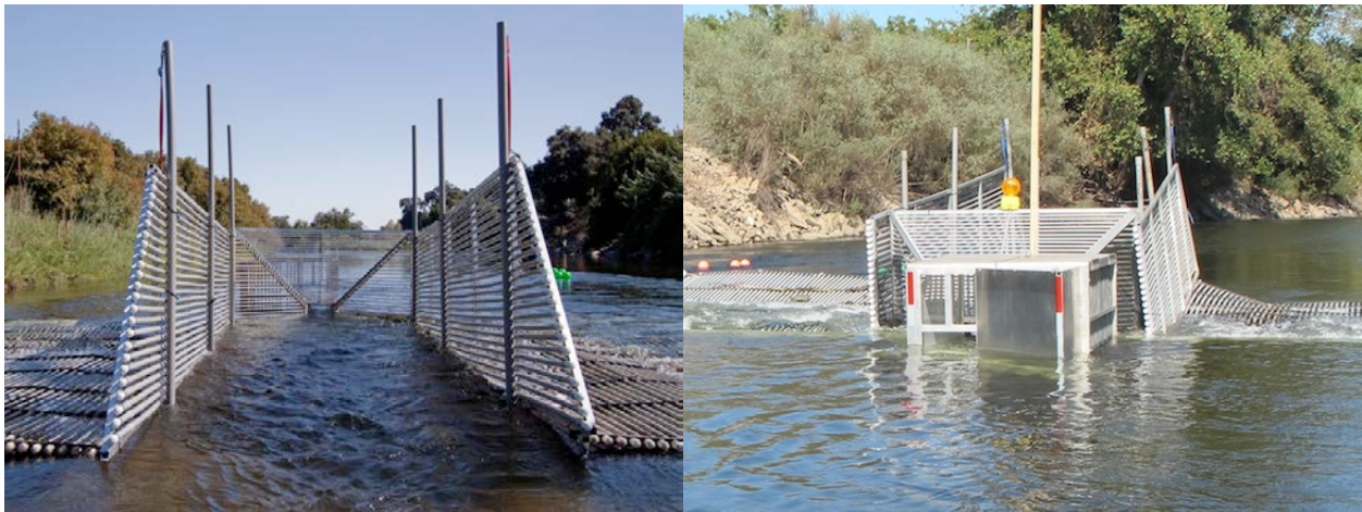
Figure 4. Left: Downstream photo of the fyke that contains Vaki system. Right: Upstream side of livebox where fish migrating upstream of the weir exit the Vaki system.
