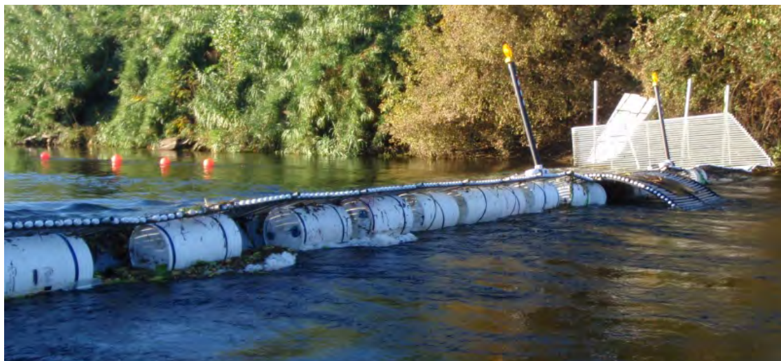
Figure 2. Photograph of the flotation barrels lining the underneath of the resistance weir.
