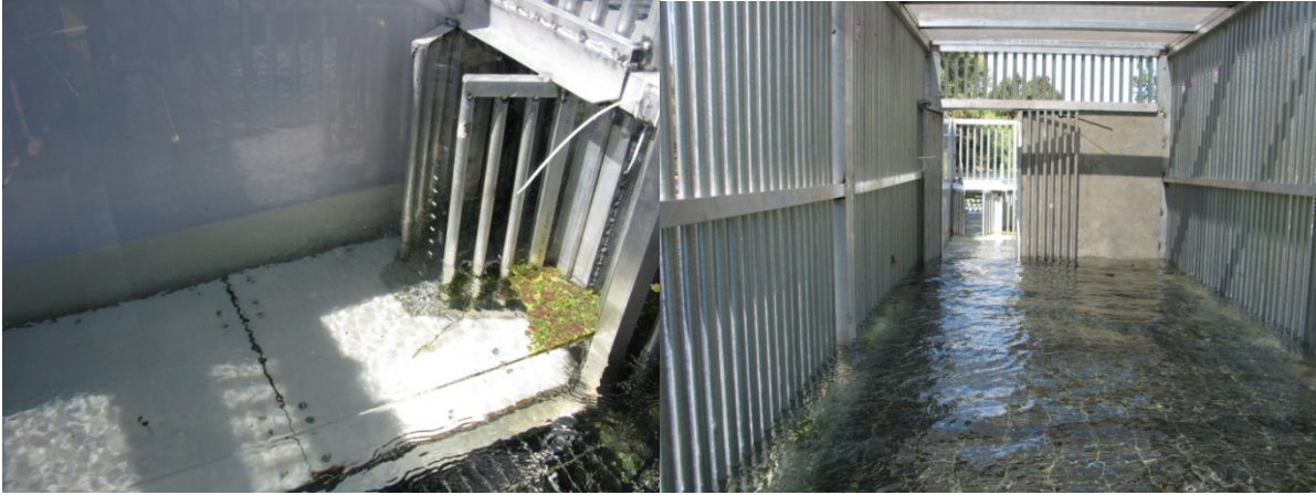
Figure 3. Left: Photograph of the fyke at the opening of the passing chute/trap. Note the fyke opens up into the viewing lane as pictured. Right: Livebox just upstream of the camera viewing lane.
