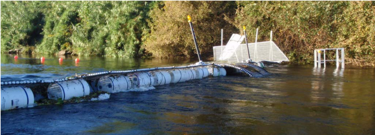
Figure 7. Photograph of the flotation barrels lining the underneath of the resistance weir.
