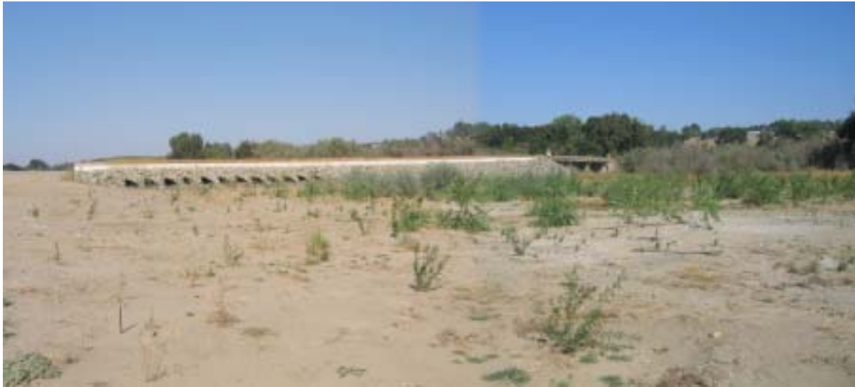
Figure 60. Series of twelve culverts in 7/11 Reach that bypasses high flows on the floodplain through the southern abutment of the 7/11 Materials haul road bridge.
